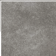
CLOSE-UP OF TILE
