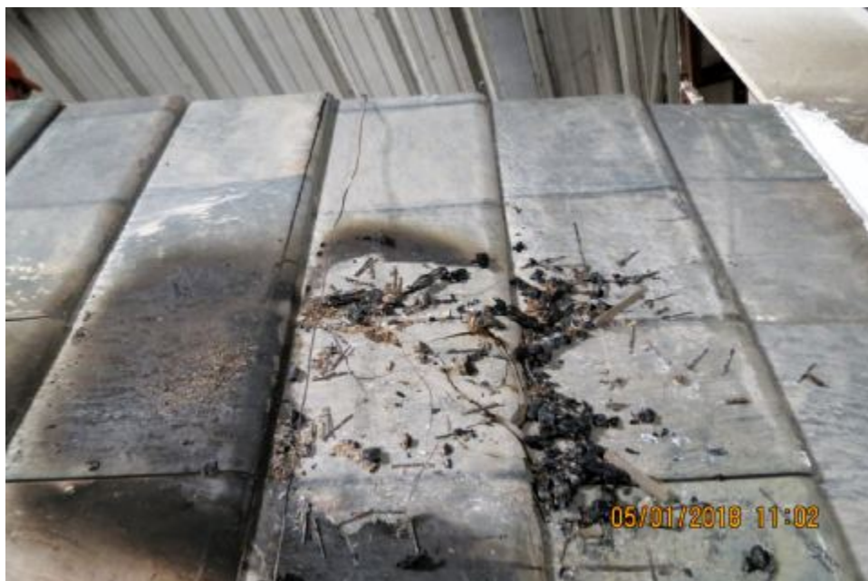
Photo No. 4 TEST #2 AFTER
